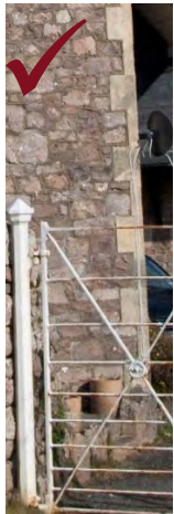
Above: traditional stone quoins (left) provide structural support to the corner of the building. This approach has been copied in a more contemporary way using engineering brick (middle) However the use of 'applied' rounded stones (right) is visually inappropriate
