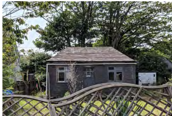
Below: Chalet at Sandy Lane
