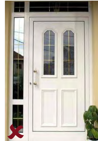
Above: poor example of doors - use of uPVC and resultant inappropriate style and details Below: good examples of doors - simple design, colour and choice of ironmongery
