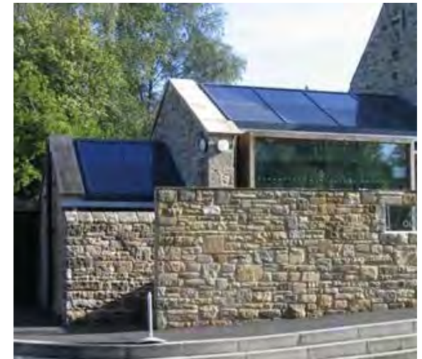
Above: PV installation integral to building design
