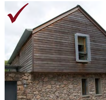
Above: attractive use of timber to upper storey of contemporary extension, with lower storey built in appropriately laid and detailed stonework visually inappropriate
