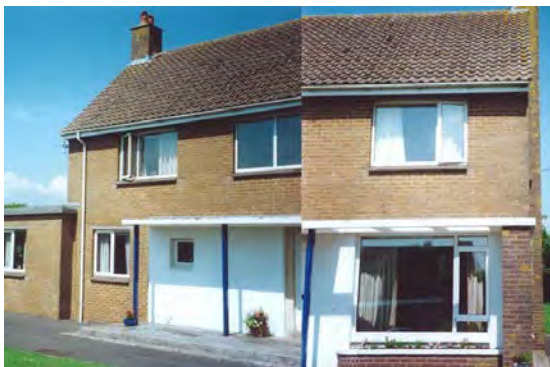
Above: before renovation
