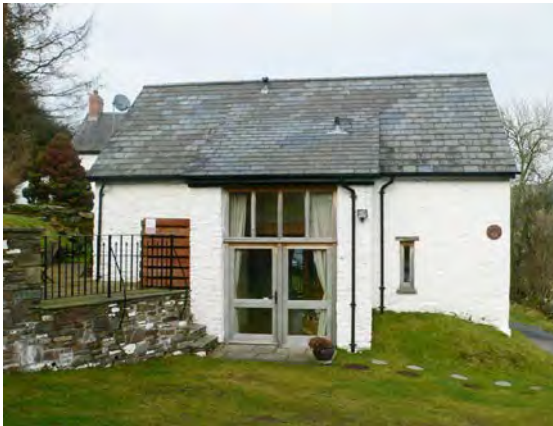
Above: existing openings retained and simply glazed to provide access and daylighting. Brecon Beacons National Park
