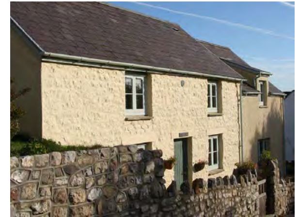
Above: Subordinate extension (right) to traditional cottage, Landimore
