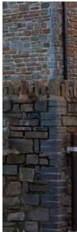
Above: traditional stone quoins (left) provide structural support to the corner of the building. This approach has been copied in a more contemporary way using engineering brick (middle) However the use of 'applied' rounded stones (right) is visually inappropriate
