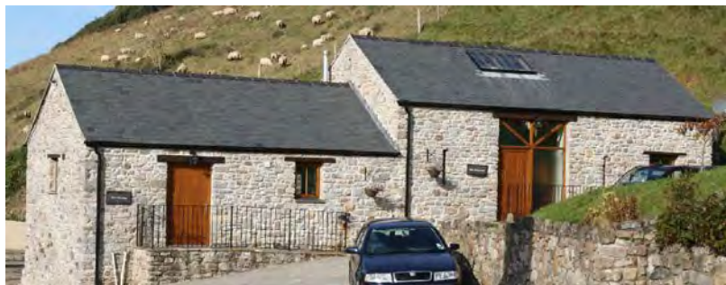
Above: Barn conversion for use as holiday accommodation, Glebe Farm, Cheriton. Utilising existing openings, simple detailing and incorporating level access.
