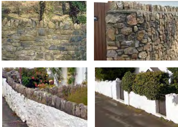
Above: appropriate types of stone walling Below: different styles of whitewash finish
