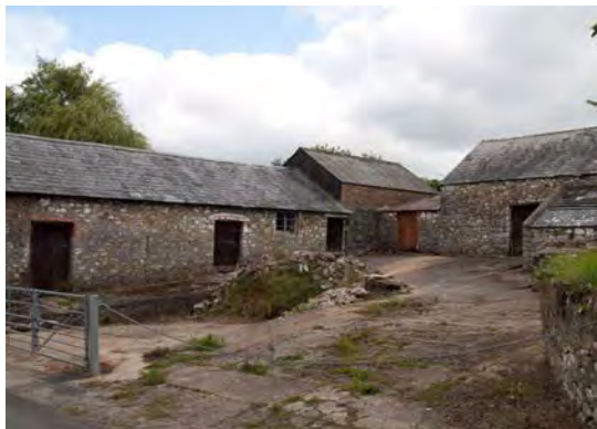
Below: farm buildings used as basis for the preparation of illustrative examples (right)
