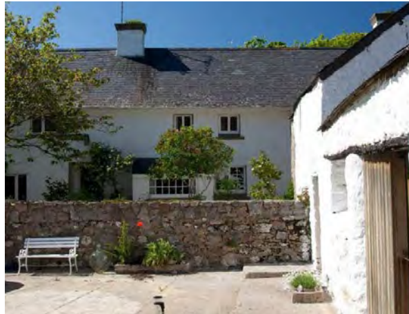
Above: Great Pitton Farm, (Grade II listed), is an example of traditional Gower Farmhouse with small windows and slated roof
