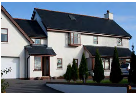
Above: after renovation
