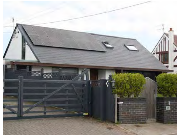
Above: Photovoltaics to roof, Southgate
