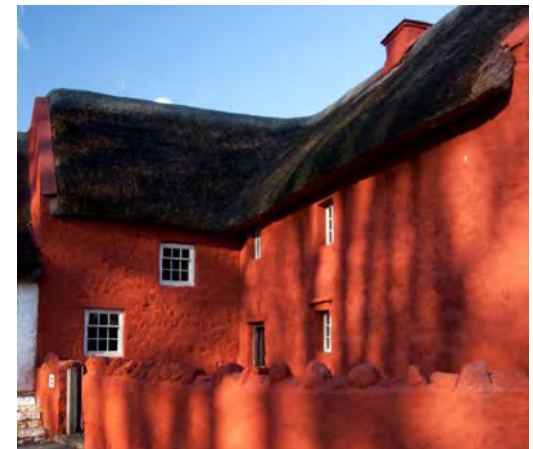
Below: Kennextone Farmhouse was originally covered with a limewash coloured with ox-blood
