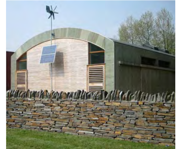
Above: Torfaen Council Eco-Building © White Design
